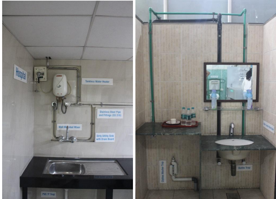
One pipe, two pipe systems.
