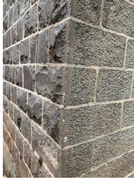
Figure 4 – Stone wall with dressing style
