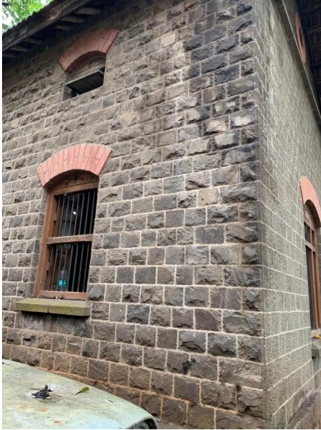
Figure 4 – Stone wall with dressing style
